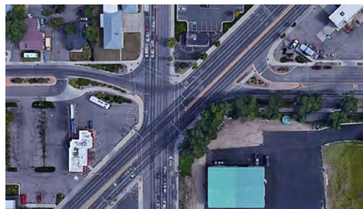
Figure 58: The South & Russell intersection.
